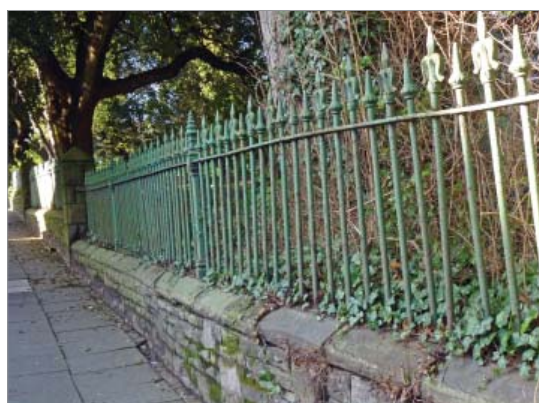
The listed railings around St James's Churchyard
