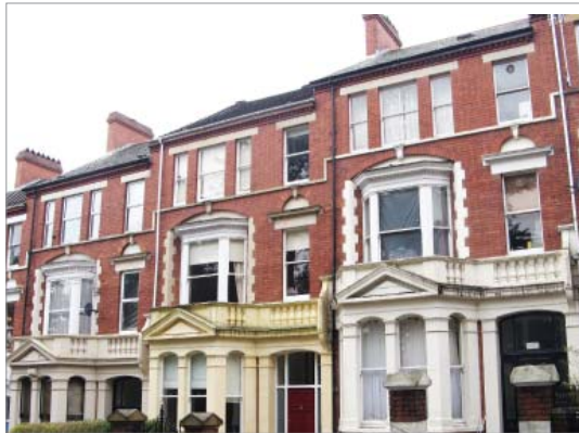
Listed houses in St James Gardens
