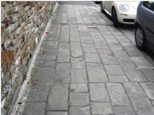
Stone paving in Richmond Road
