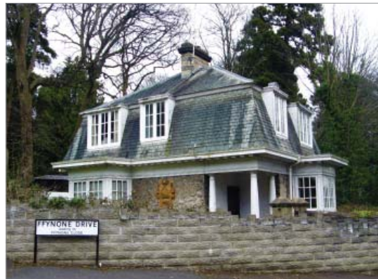
Entrance lodge to the Mansion House, Ffynone Road
