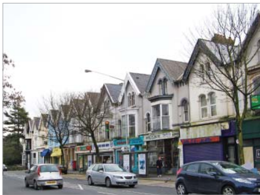
Uplands Crescent south side
